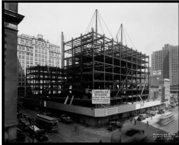
Image 4. A photo of the Chrysler Building's early construction 55
