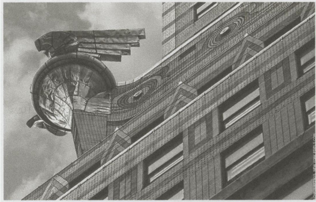
Image 6. A photograph of the stainless-steel automobile themed decorations on the building 57
